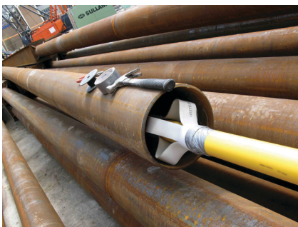
Figure 2. Centralizers in pipe pile section.
