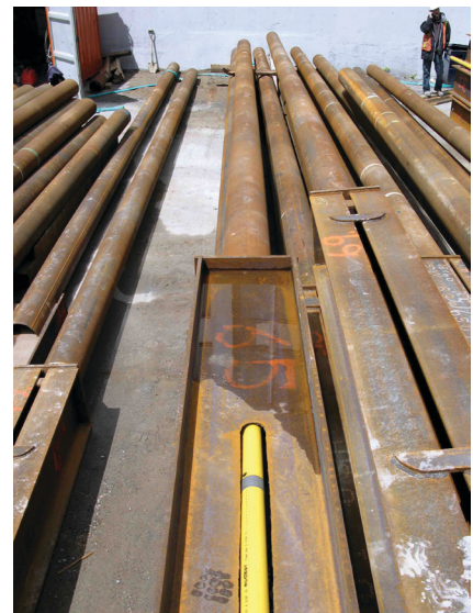
Figure 1. Lower section of pile with inclinometer casing transition to pipe pile.
